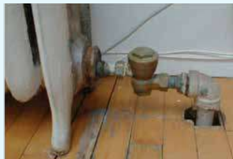
Figure 5: In-Unit Steam Trap
