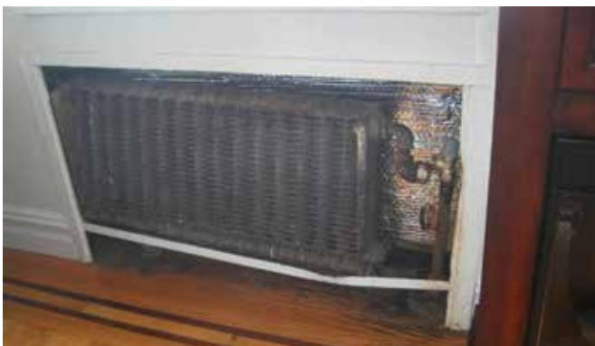
Figure 8: Radiant barrier installed
