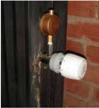
Figure 10: 1-pipe steam TRV
