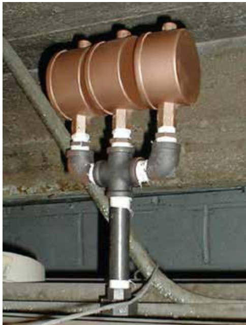
Figure 4: Steam Venting
