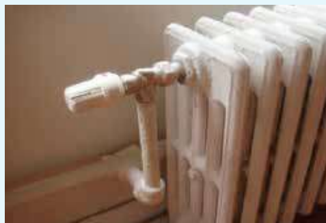
Figure 5: Two-Pipe Steam Thermostatic Radiator Valve (TRV)
